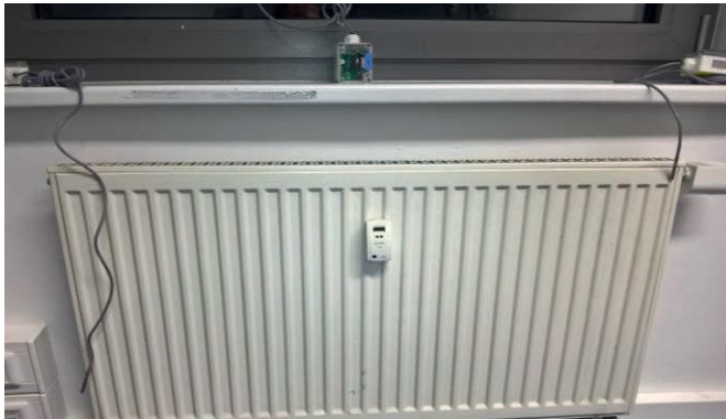
Figure 4: Measurement points at radiators
